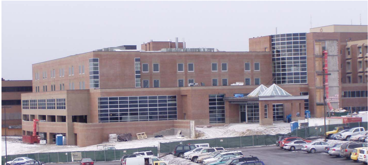
Photograph 3: View from South-East showing the brick façade and curtain walls
