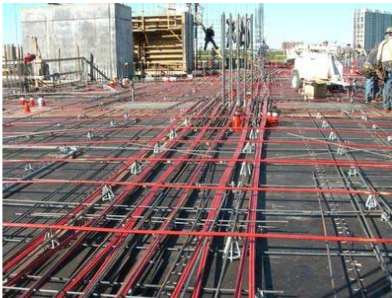
Figure 9: Post-Tensioned Slab
